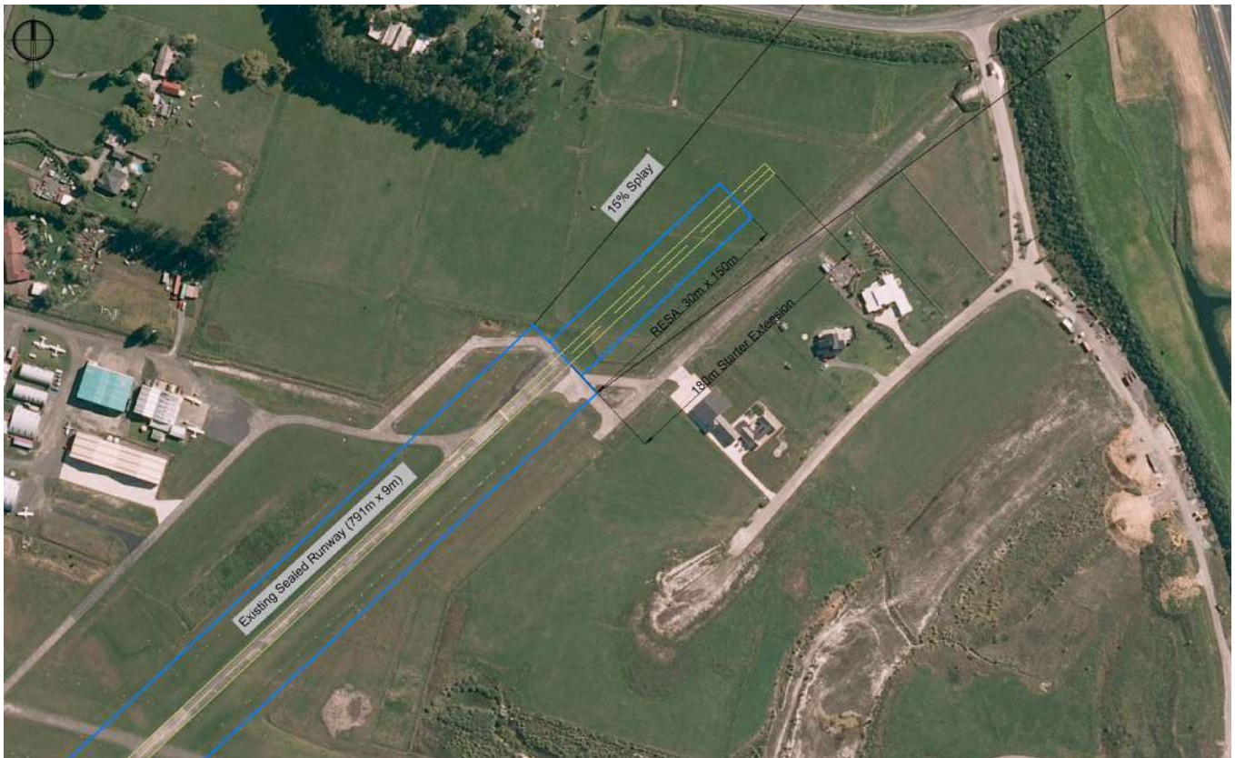
Stage One runway extension
