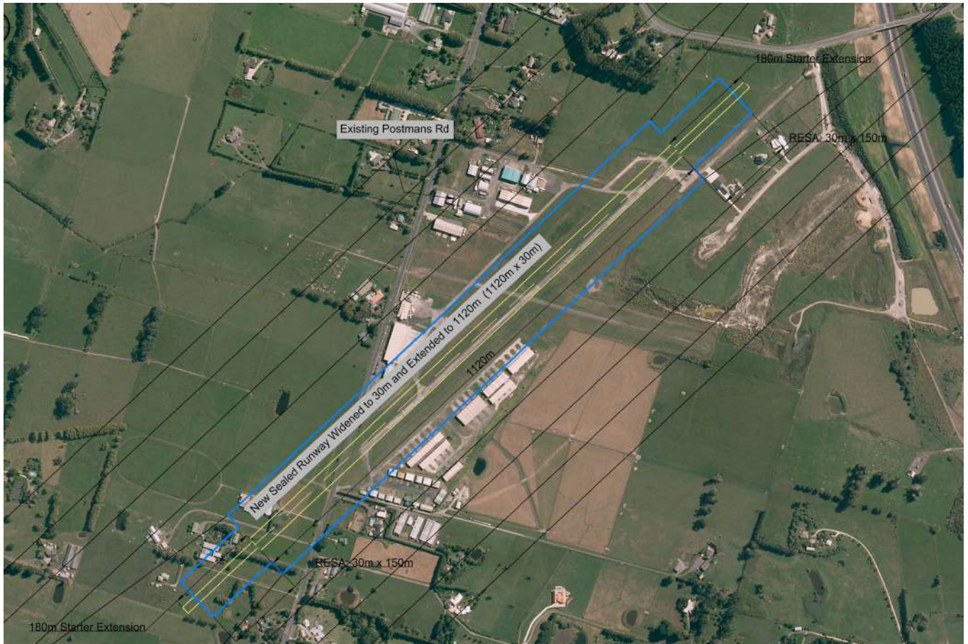
Stage 3 runway extension
