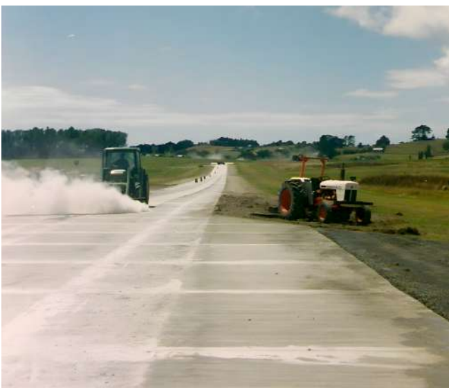
1990's - New concrete runway nearing completion
